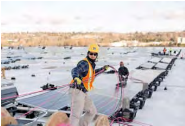
Rooftop solar installation on the IKEA in Renton, Washington. Photo courtesy of A&R Solar.
