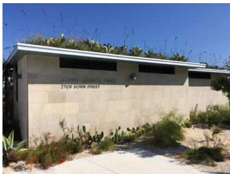
The clubhouse of John Gaines Park in the Mueller development features a green roof and rain gardens.
