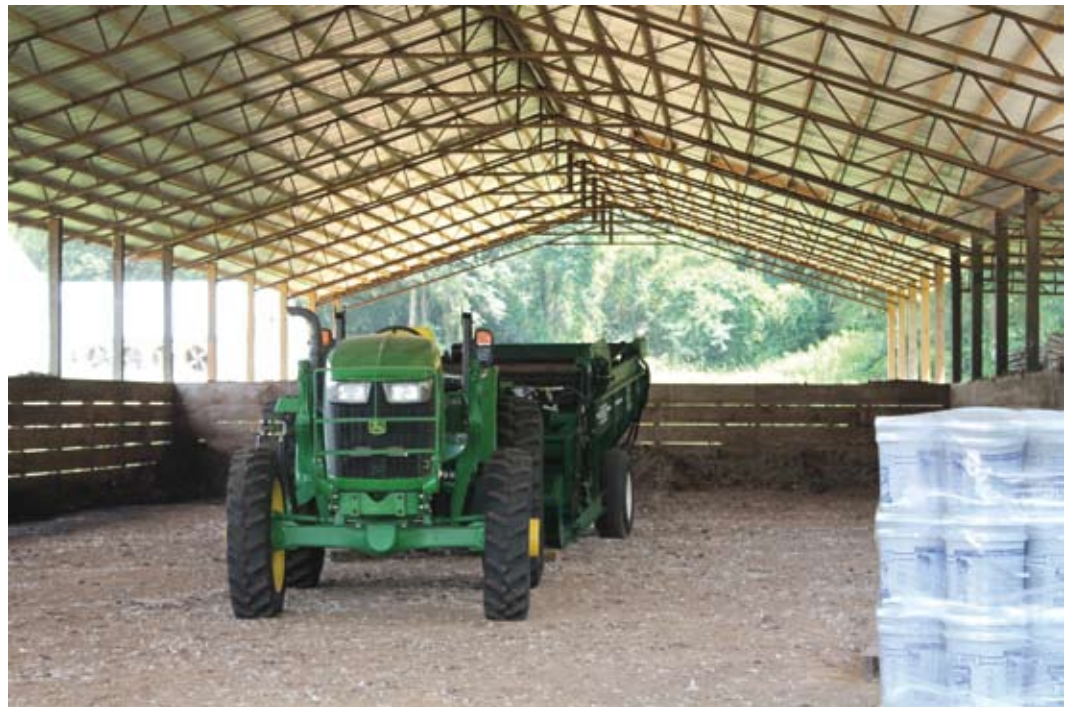
Construction of this poultry litter storage facility in Hazlehurst, Mississippi, was funded by the USDA’s Environmental Quality Incentives Program. Photo: Judi Craddock, USDA NRCS via Flickr, CC BY 2.0.
