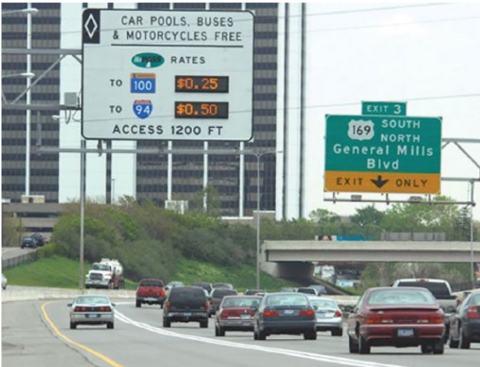
A growing number of cities are using high occupancy/toll lanes as a tool to manage congestion. Photo credit: Federal Highway Administration
